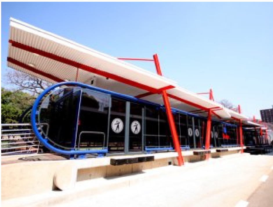
Figur 6. BRT-station Rea Vaya-systemet i Johannesburg, Sydafrika. Foto: www.engineeringnews.co.za
